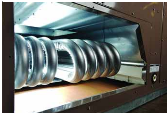
Figure 16: Bottom Supply Opening For Side Duct Conversion
