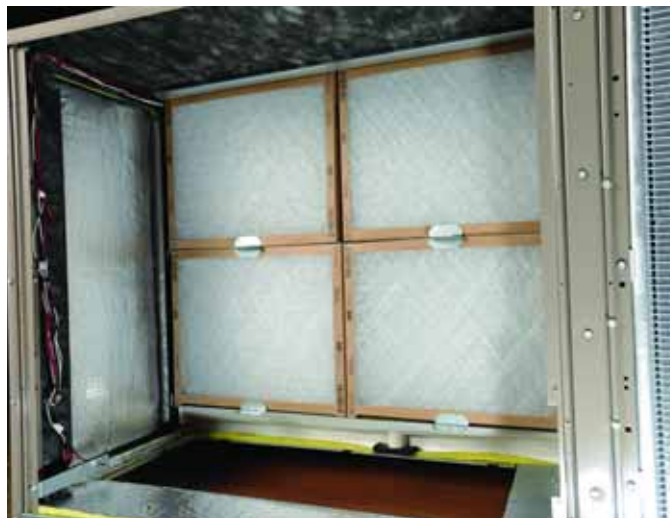
Figure 15: Bottom Return Opening For Side Duct Conversion
